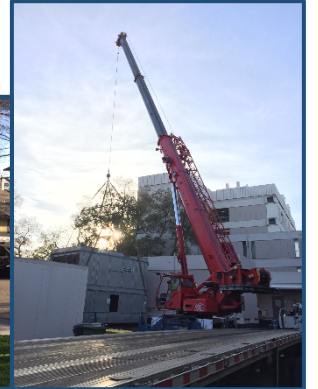
"New" Chiller and Tower Repurposed from campus
